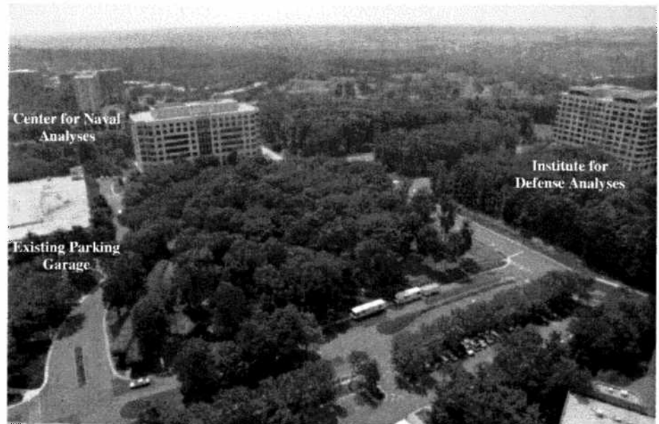
EXISTING MARK CENTER VIEW OF PROPOSED ARMY BRAC 133 SITE
