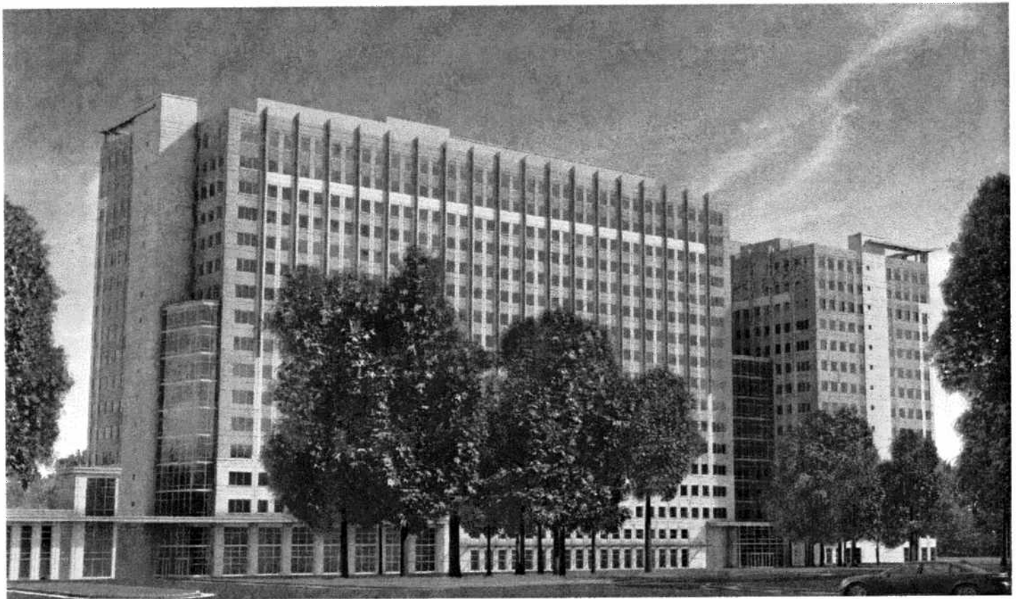
EAST TOWER (Foreground) AND WEST TOWER (Background at Right) BUILDING DESIGN AS VIEWED FROM NORTH PARKING GARAGE SIDEWALK
