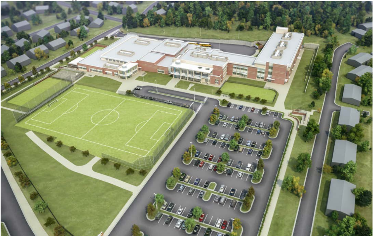
Aerial view looking east
