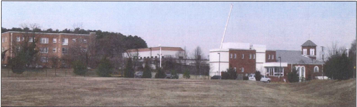
Area B (between King Street and Oakland Baptist Church)
