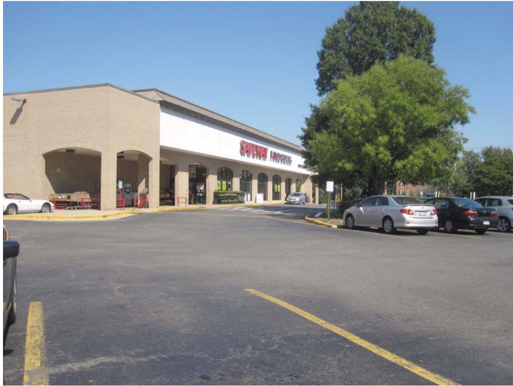
Figure 20. View along south elevation of Safeway (3526 King Street) looking southeast across the parking lot.
